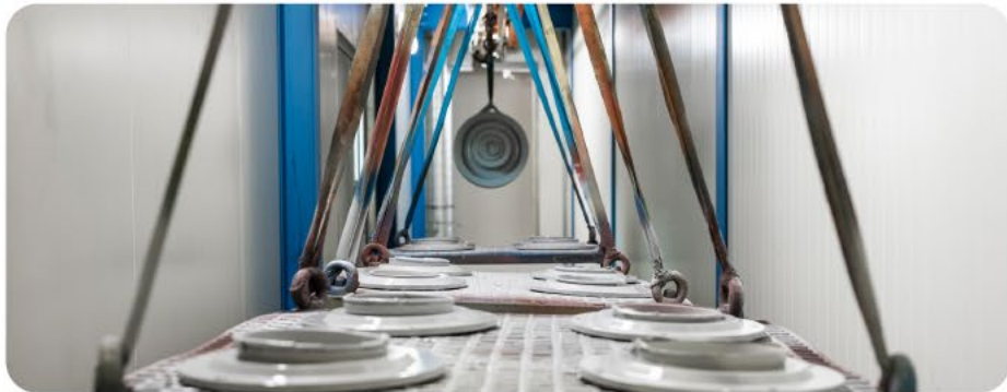
View into the semi-automated drying plant with reduced heat output and heat recovery
